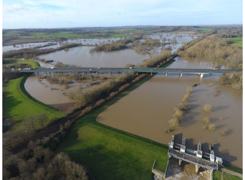
Photo of the railway line running through the Leigh FSA during impoundment, Feb 2020
